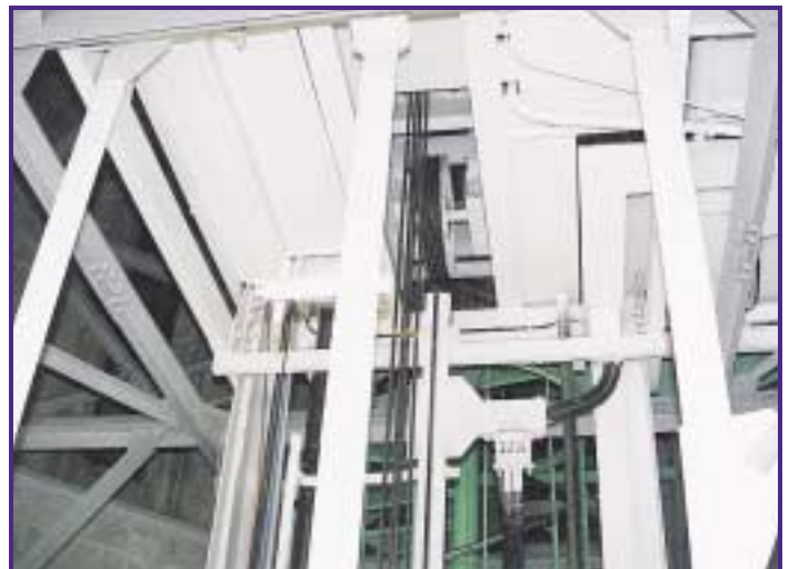
Detail shaft top
