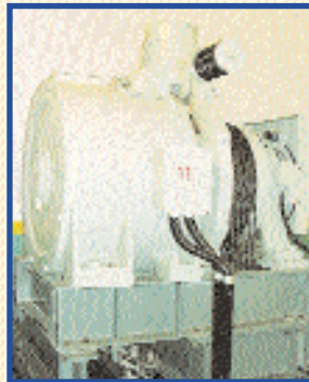
AC gearless machine (service lift)
